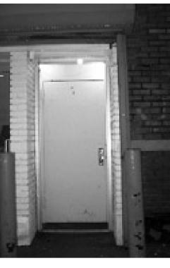
door askew out of frame, lock difficult to turn aluminum threshold 10" to rear door metal rear door 6' 10 7/8" x 2' 1 13/4" rear doorframe 7' 2" x 3' 41/2" round rear doorknob at a height of 3' 1", diameter 2 3/4"
